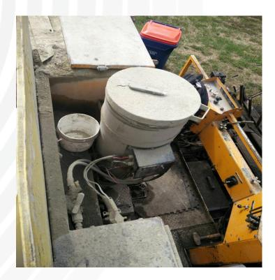
Slurry Fil fibers being added on Aggregate belt prior to discharge in Mixer box.
