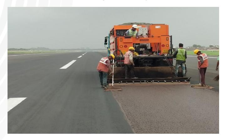
First project in India, where highly modified Micro surfacing with fibres was executed on an active runway at Ahmedabad Airport Sep 2018 of AAI.
