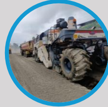
Pulverization of soil with Recycler
