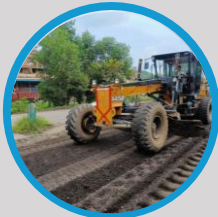
Grading & Profiling with motor Grader
