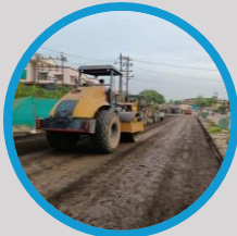
Compaction by Soil Compactor
