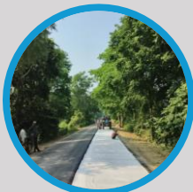
Laying of Paving fabric and Providing BC / PQC over the stabilized Layer
