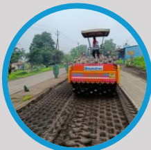
Compaction by Pad Foot Roller
