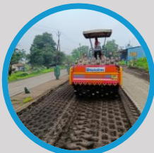
Compaction by Pad Foot Roller
