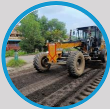
Grading & Profiling with motor Grader
