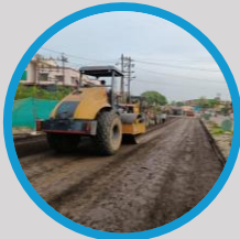
Compaction by Soil Compactor
