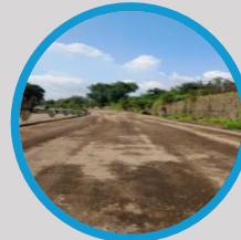
Final surface after Compaction
