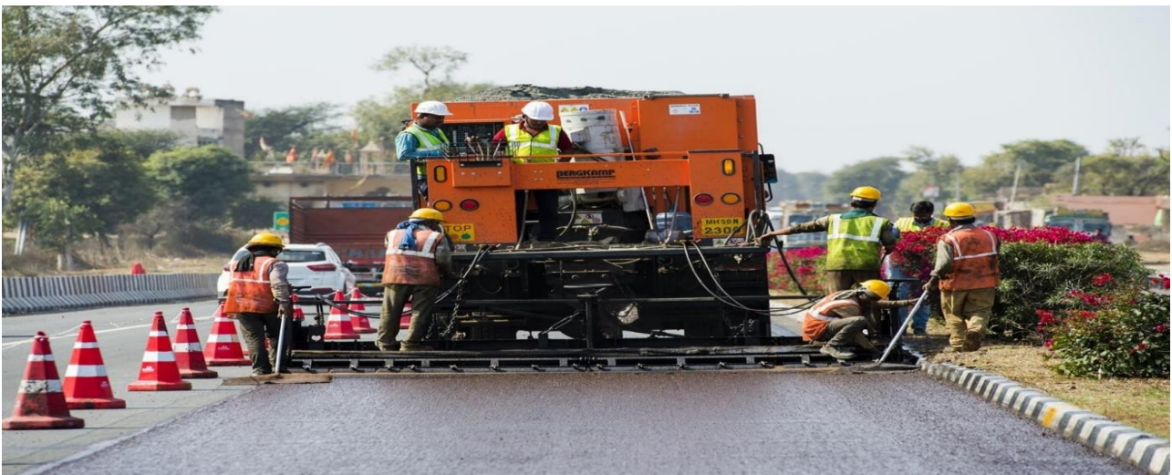
Figure 7. Microsurfacing
